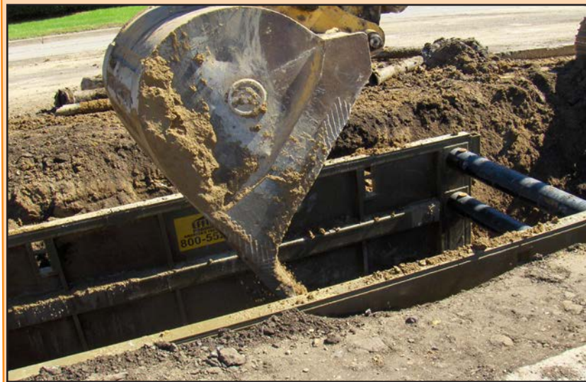
Without a trench shield, the slope required for this excavation would close most of the road and adjacent sidewalk.
