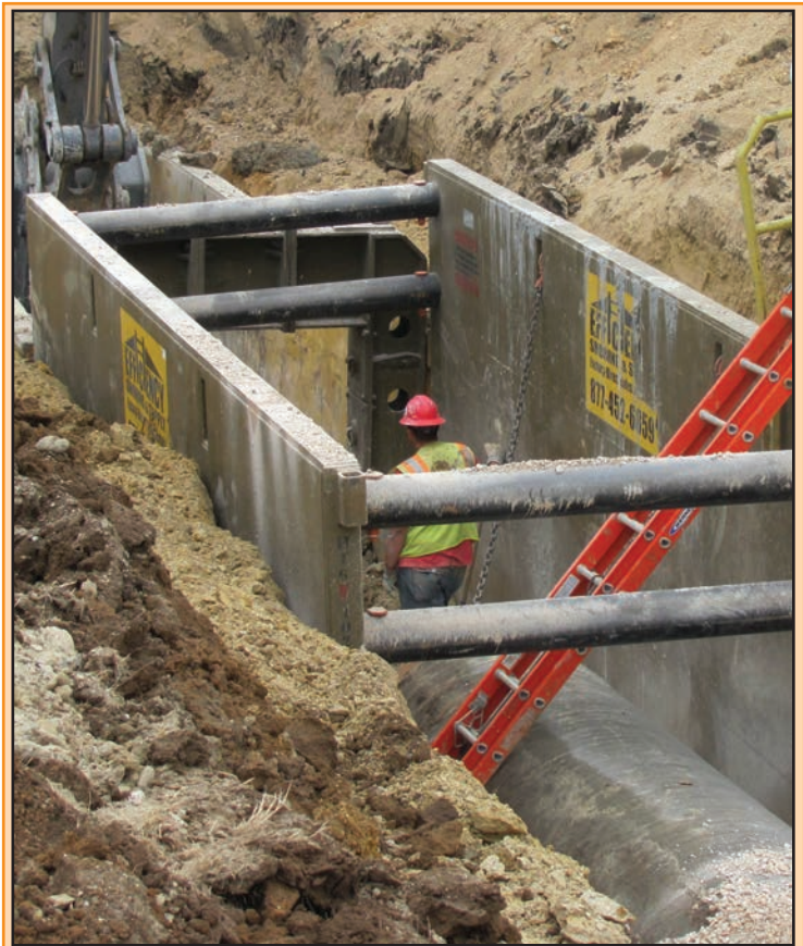
When installing a new water main across rural Texas, nothing prevented this contractor from open-cutting and sloping...except the time and money needed to excavate the excess dirt.
