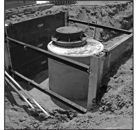
Two-sided configured with long spreaders for manole installation
