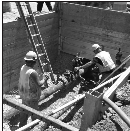
A three-sided configuration with end panels pinned 305 mm up in corner posts allowing gas utility to run through
