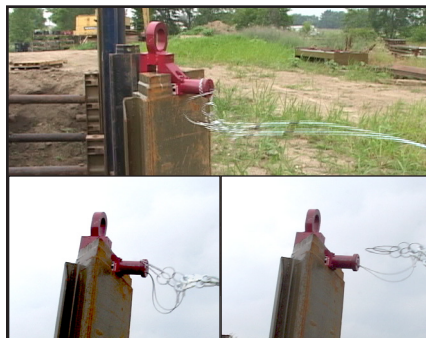
7. After positioning and securing the component, release the safety ring by pulling the release rope/line.
