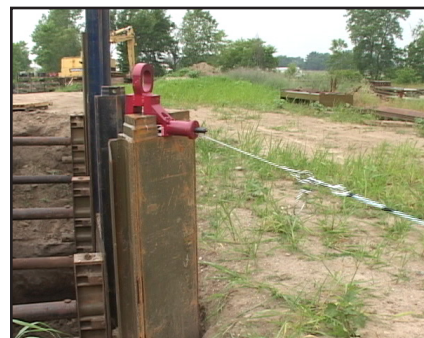
8. Then pull on the release cable to free the Shackle from Component lifting lug.
