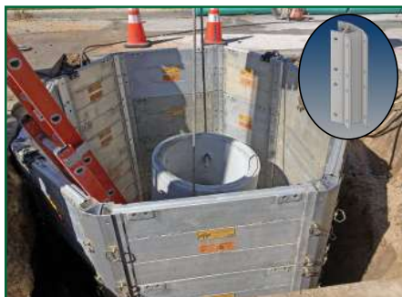
Octagon Configuration w/ 135° Corner Posts
