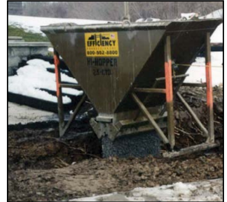
Hi-Hopper in Use
